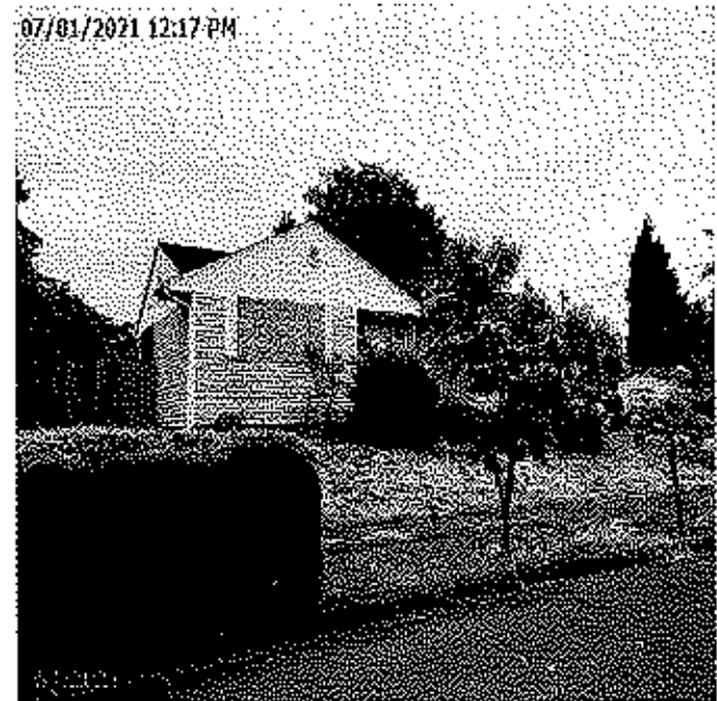
Address: 11312 NE DAVIS ST. PORTLAND OR 97220 Date Completed: 07/01/2021 Description: SIDE VIEW
