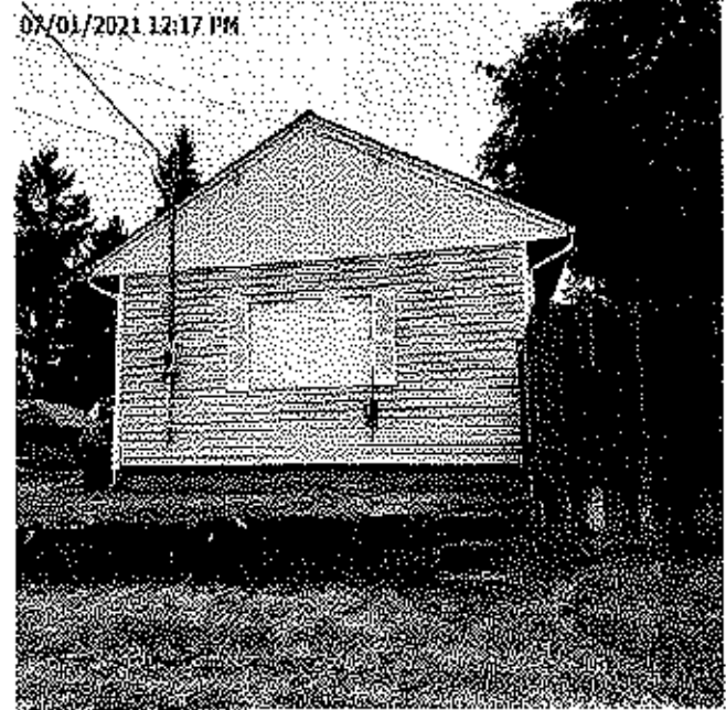
Address: 11312 NE DAVIS ST. PORTLAND OR 97220 Date Completed: 07/01/2021 Description: SEEB VIEW
